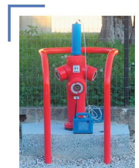
Fire hydrant injection
